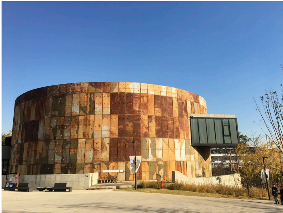
Fig. 13. Remodeled and existing rusting oil tanks performing as containers for various cultural content. Culture Tank. (Source: author's photograph, 3 November 2018).
