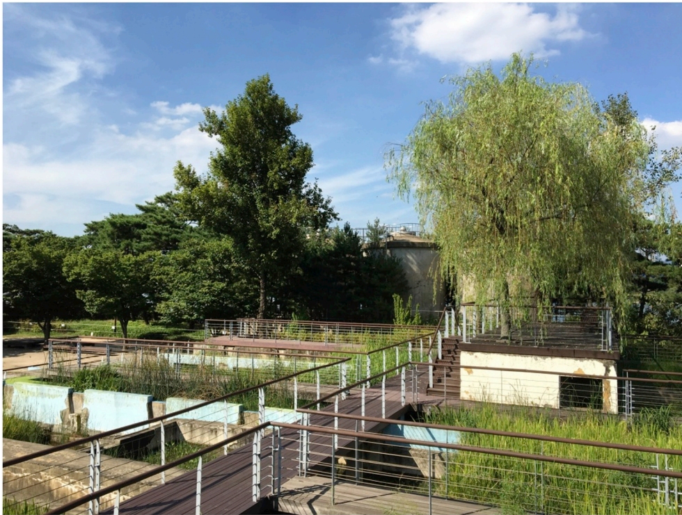
Fig. 3. Industrial structures of a settling basin for chemicals now functioning as a nest for aquatic ecological processes. Seounyudo Park. (Source: author's photograph, 22 August 2018).
